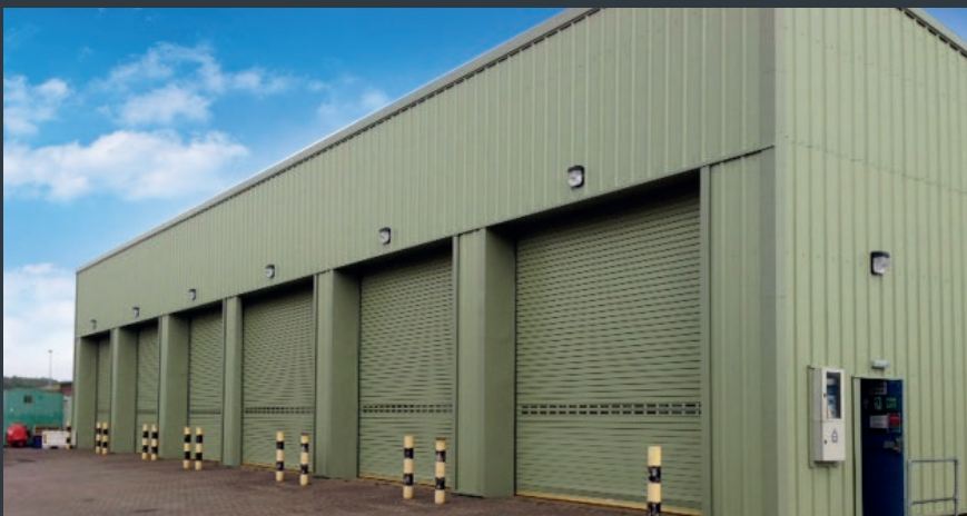
RAF Wittering, Insulated Roller Shutters using ATEX certified motors.
